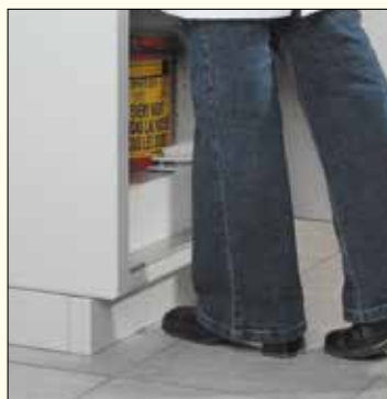
Base set back to prevent people from hitting their feet on it.
